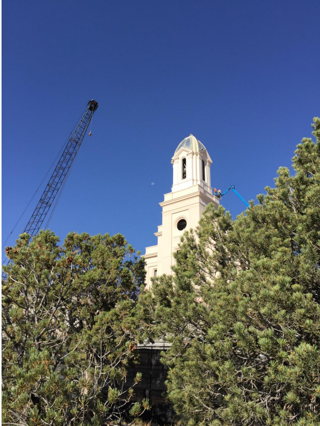
Cedar City Temple, after steeple was installed.
